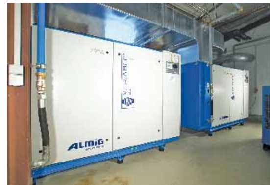
Two speed-controlled, air-cooled screw compressors of type VARIABLE 35
